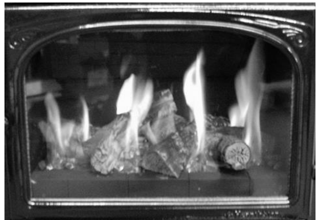
Figure 34 – Typical Burner Flame Appearance
